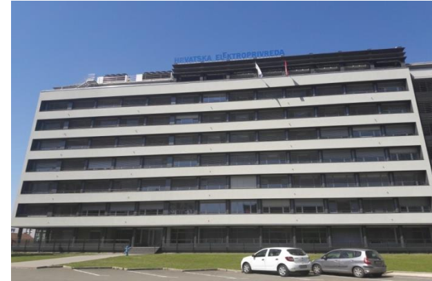
Fig. 1b. Building B
