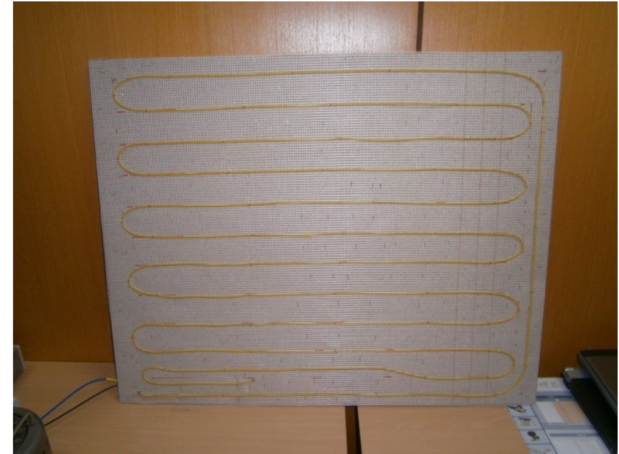
Figure 8. Detail of installation of the modify LTEFHP
