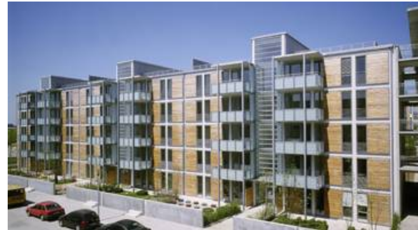
Housing development in Munich-Riem WA1 http://www.herzog-und-partner.de/english/projects/projects-riem_wa1.html
