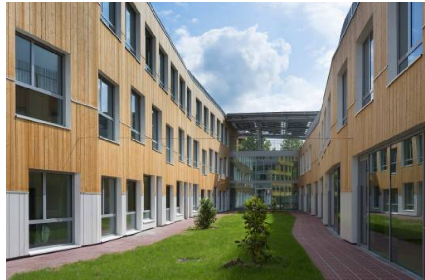
Zero Energy school in Saint-Ouen, France http://www.archdaily.com/459482/zero-energy-school-mikou-design-studio/
